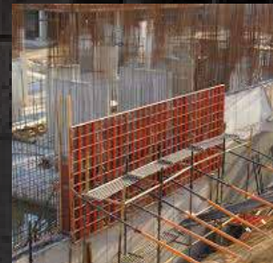
Retaining Wall Formwork
