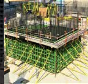
Retaining Wall Formwork
