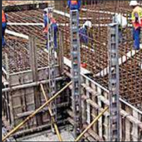
Column Formwork
