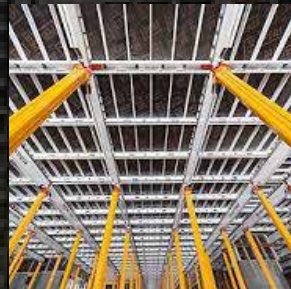
Slab Formwork
