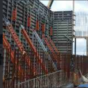
Wall Formwork
